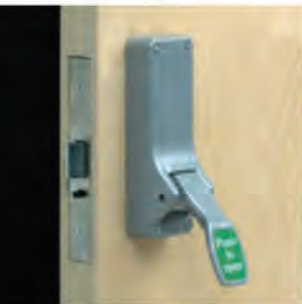
Emergency exit device on door
