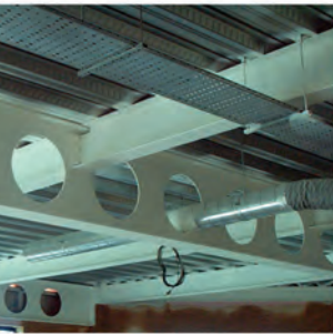
Cellular beam coated with intumescent paint.
