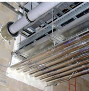
Correctly installed penetration seals. Courtesy of Siderise Ltd.
